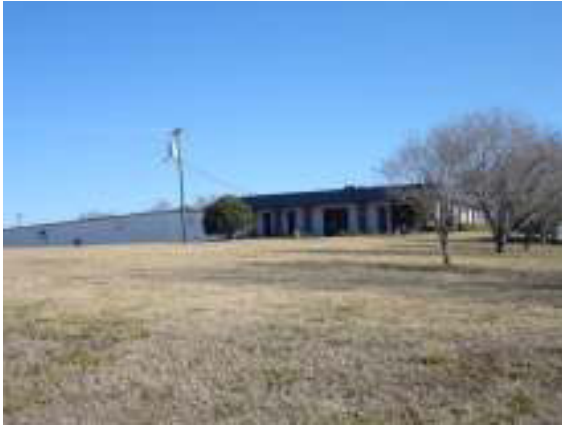
Industrial building to the east.
