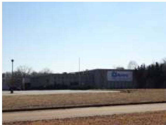
Aurora Specialty Textiles building to the north.
